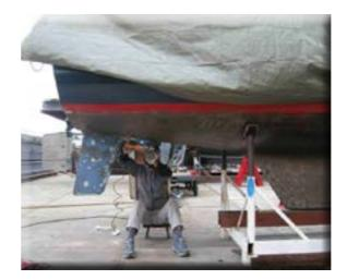
It was then treated with HP-E45KL, Thixotropypowder HP-PK22 and Microballoons HP-MB2. To increase the strength and durability. a Glass Fabric "Silane" (HP-VJ50C) was laminated with HP-E45KL.
