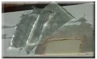
Laying out the reinforcement fibers on the surface
