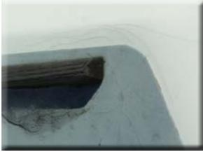
Cracks and holes in the gelcoat
