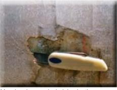
Massive damage incl. delamination, Area must be rebuilt with fiberglass fabric or scrims
