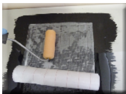
The peel ply absorbs excess resin. A deaeration roller for careful impregnation should be used.
