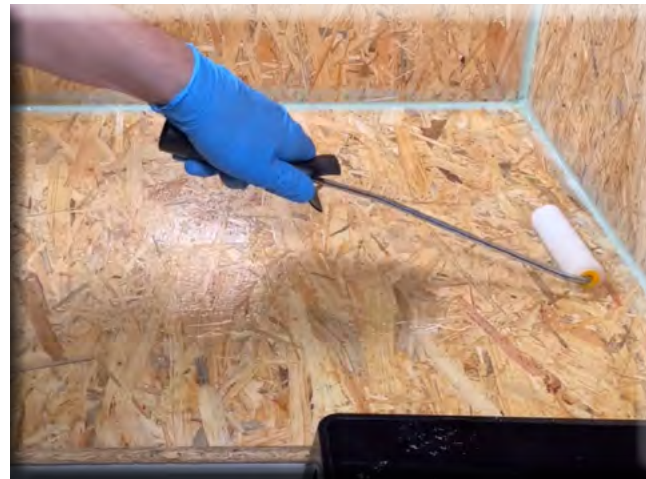
Application of the epoxy resin system
