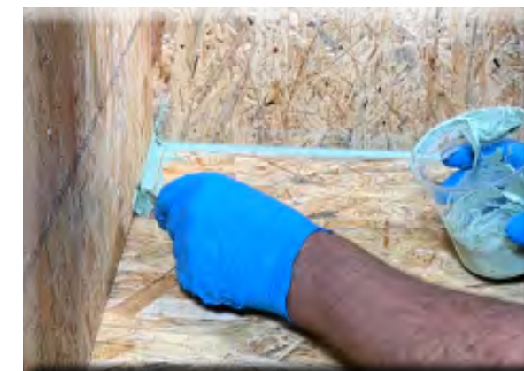
Applying the epoxy putty
