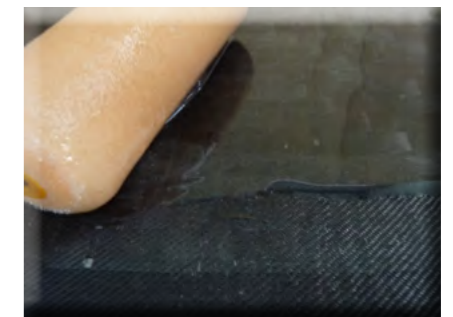
Epoxy resin is distributed with flocked foam roller
