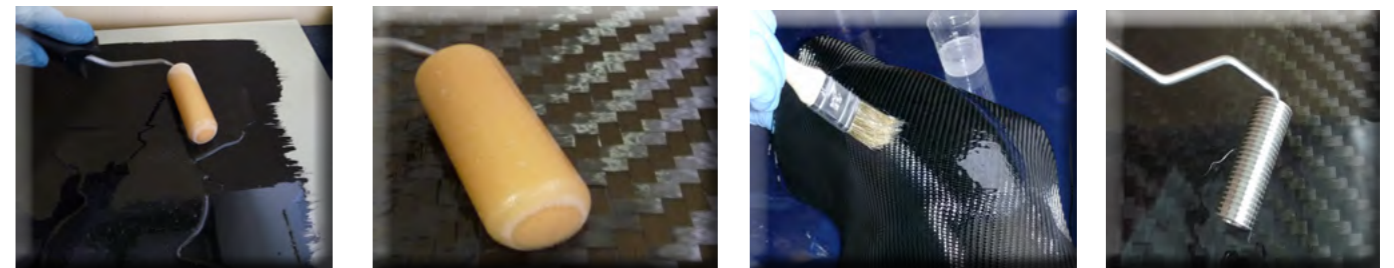
The epoxy laminating resin is applied with a flocked foam roller or brush. The fabric is then applied and thoroughly saturated. Air bubbles are removed with a deaeration roller.
